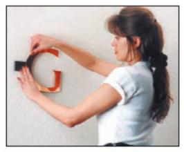
Push the letter into the drill holes using a shim to assure the proper standoff of the letter from the wall. Repeat steps 3 through 5 for the rest of the letters.
