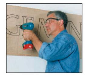
3. Mark holes with center punch, then drill 1/4" holes 3" deep where indicated on your template. Remove the template and clean out all drill holes using any of the following methods: a quick puff of air; using the vents on your drill; compressed air or a turkey baster
