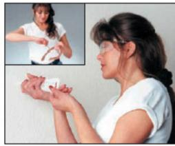
4. Insert the studs into the stud holes on the back of each letter. Place letters in holes on wall before applying silicone to verify position. Adjust as necessary, now fill the drill holes in the wall of the first letter with silicone.
