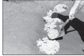
Lay down a bed of sand approximately 1/2" thick on ledge of pond and rake smooth. The top of ledge should be at water level. Smooth the sand, make certain the surface is level.
