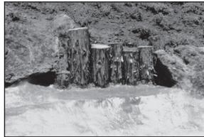
Mark the water line with a string line and cut a ledge 4" to 6" below the water line. This provides an edge where the stumps appear to be holding back the water. Glass the wall behind the stumps and
