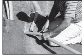
Lay a 2" diameter mailing tube, cut lengthwise and in sections, to form the curve at the edge of the pond. This creates a uniform raised edge which keeps drain water and debris out
