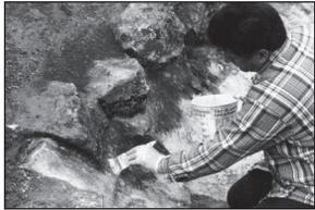
Lay fiberglass pieces around the perimeter rocks. Lay larger pieces (up to 18" x 18") toward the bottom of the pond. Check water line as you proceed around perimeter. Construct edges to keep rainwater from draining into pond.
