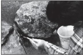
Use the bristle ends of a brush, poking rather than brushing to work mat into place and blend pieces together. A two or three inch wide brush is good for small or irregular areas.
