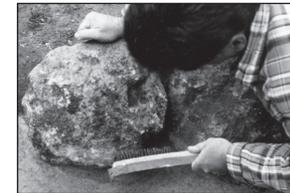
Wire brush rocks from waterline down to ensure the adhesion of the fiberglass to the rock. Glassing over moss, dirt, or slag will impair adhesion and a waterproof seal. There is
