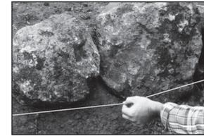
Use a chalk line to provide reference points to determine glassing height on the rocks. Determine the water line by the height of the waterfall and the area where the filter will be constructed.
