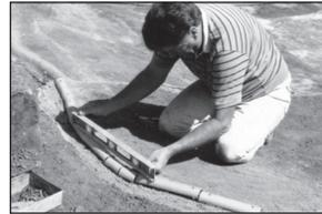
Hold tube sections in place by driving 3" or 4" nails through the cardboard tubes into firm ground. Raise or lower the tubes on the nails and level before laying the fiberglass mat. Provide a covered surface by
