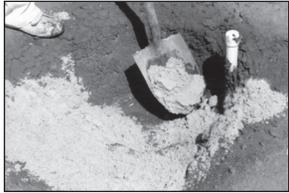
Areas needing special attention in and around a pond are the low places, the sump holes which may have pipes or wires going through the fiberglass, ledges for plants, and depressions for large rocks. Cover all of these areas with a thin layer of damp sand, creating a smooth surface with gradual curves. Connect the sides and bottom of the sump hole in this manner. Put the submersible pump at the lowest point of the pond for easy cleaning and to protect the pump from running dry.
