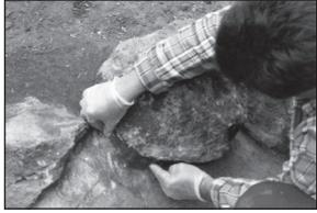
Cut small strips of fiberglass mat (approximately 6" x 8"), saturate with resin and lay them in place bridging the rock onto the dirt and sand base. Two layers of mat are advised in irregular rock-dirt areas. Wet the fiberglass mat on a clean working surface and place pieces tangent to the bridging surfaces. Overlap adjacent pieces 1" to 2".
