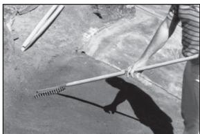
Create a uniform rim for edges of the pond that will border lawn, ground cover, gravel, cement, or other materials. Make this division by cutting a ledge, about 10" to 12" wide, at the water line.
