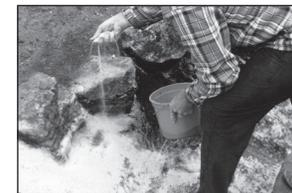
While this final color-coat is still wet (within 10-15 minutes of the mix), dull the surface to make it look more natural by sprinkling dry washed sand onto the wet resin surface. Be generous with the sand. After the resin cures, sweep off excess sand and reuse it in other areas. The finished waterproof shell will withstand radical temperature changes and earth movement—unlike most do-it-yourself concrete ponds.
