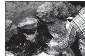
After thickened and pigmented resin is brushed on the cured fiberglass surface, carefully examine the surface to look for potential leak areas. If an area is spotted that looks resin-starved or is not reinforced enough, cover with a piece of mat, overlap the surface by 2", wet-it-out, and blend into the rest of surface. Sand rough areas before patching. A disk grinder is recommended for large ponds.
