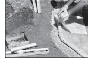
Saturate fiberglass pieces with resin at your clean working surface and carry immediately to pond edge. (A movable working surface in center of pond is a time-saver.) Pieces larger
