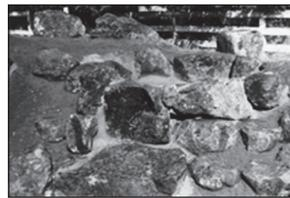
After packing and settling the berm, soak the loose dirt to compact it for a firm support base for heavy rocks. Use mortar to bed the main rocks that form the waterfall. (Note mortar joints on the larger rocks.
