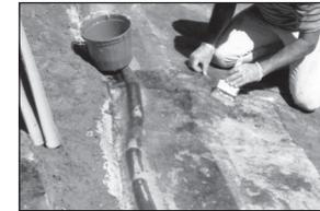
Place 2 or 3 wet pieces side by side (overlap pieces approximately 2"). Next start second row and work towards center of pond. With a brush (wet with resin), coat top surface of mat thoroughly by saturating it
