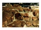
After packing and settling the berm, then soak the loose dirt to compact it for a firm support base for heavy rocks. Use mortar to bed the main rocks that form the waterfall. (Note
