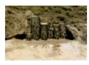
Mark the water line with a string line and cut a ledge 4" to 6" below the water line. This provides an edge where the stumps appear to be holding back the water. *Glass* the wall
