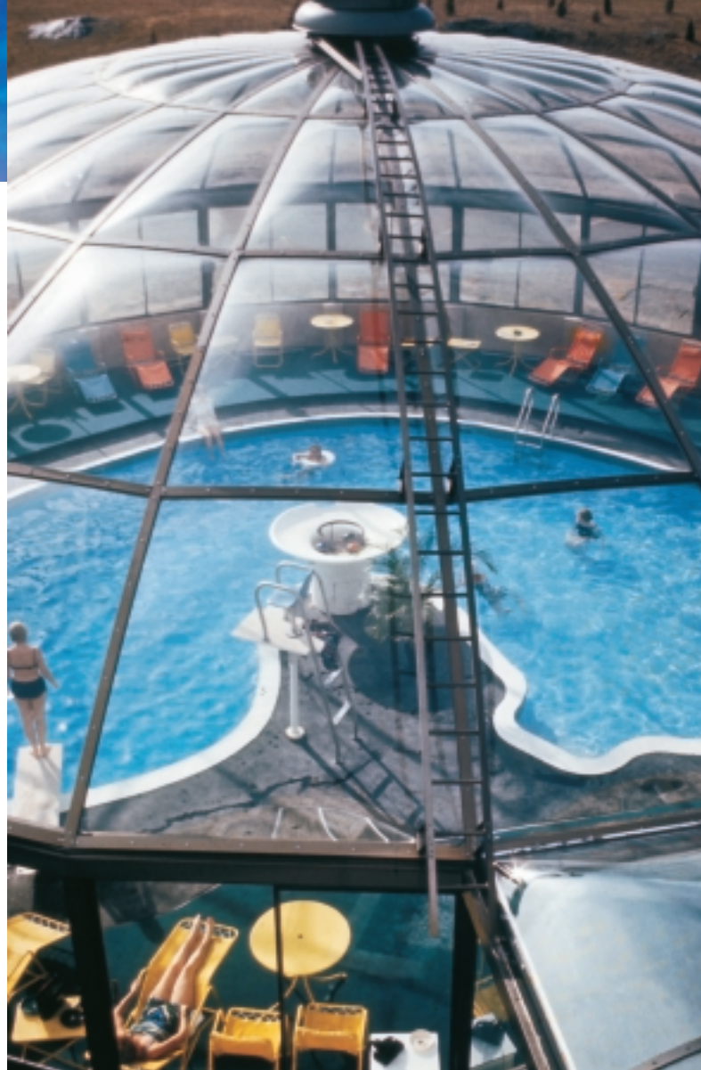
Acrylic sheet was used to create this pool cover providing architectural style and lots of natural light.
