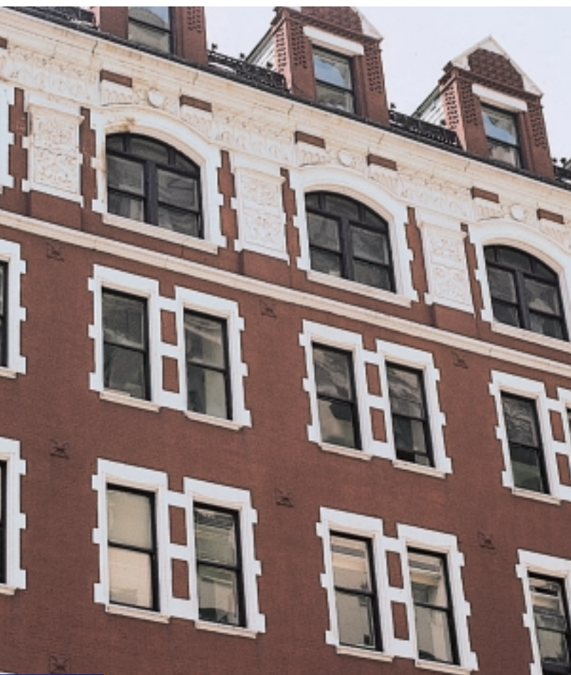
Acrylic sheet was used to retrofit this building's windows.
