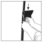
cutting the film as you go, then move the knife and tool down the edge of the window together. This will trim the film in a straight line and leave a  $^{1}/_{16}$ " gap between the film and the window frame. Repeat for the other edges.
