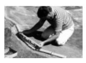
Hold tube sections in place by driving 3" or 4" nails through the cardboard tubes into firm ground. Raise or lower the tubes on the nails and level before laying the
