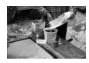
Thicken final color coat of resin with TAP Cab-O-Sil. The consistency of this mixture should be creamy enough to hang on a vertical surface and to fill
