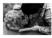
Wire brush rocks from waterline down to ensure the adhesion of the fiberglass to the rock. Glassing over moss, dirt, or slag will impair adhesion and a waterproof
