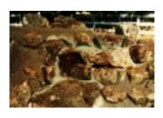
After packing and settling the berm, soak the loose dirt to compact it for a firm support base for heavy rocks. Use mortar to bed the main rocks that form the waterfall. (Note
