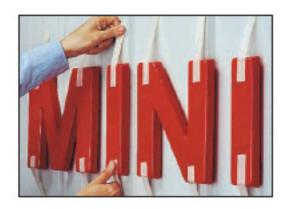
3. Adjust as needed; push letter against wall to insure good adhesive bond. Continue with the remainder of the letters, and allow the silicone to cure for at least 10 minutes before removing the masking tape. However, we recommend overnight curing for most conditions and silicones.
