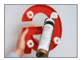
Apply silicone to all of the pads on the first letter. Position the letter on the wall where indicated on the spacing tape. Tape the letter to the wall using several strips of masking tape.
