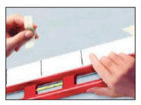
I. Clean the installation surface first. Position the spacing tape on the wall and secure one end with masking tape. Unroll, level and tape the other end. Spacing tapes show the general position of each letter only and are available free upon request.
